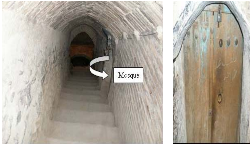
Figure10. (a) A public Nilab in Kouhpayeh to reach underground qanat tunnel for water consumption. A mosque has been located in the middle of steps. (b). Mosque door inside Nilab.
