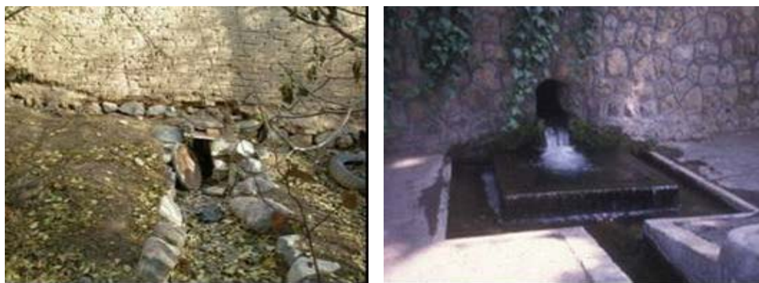
Figure 7. (a) The stream of qanat flows through inside home landscape and then is diverted into farm irrigation channels. (b) Masonry mouth of a qanat in Kohpayeh.
