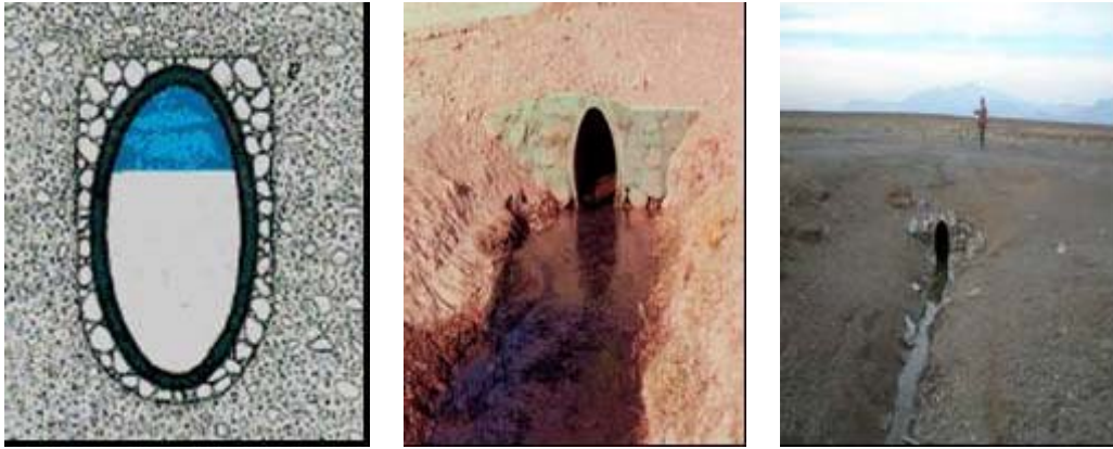
Figure 4. Kouhpayeh tunnel walls have been strengthened with tile hoops in downhill end.
