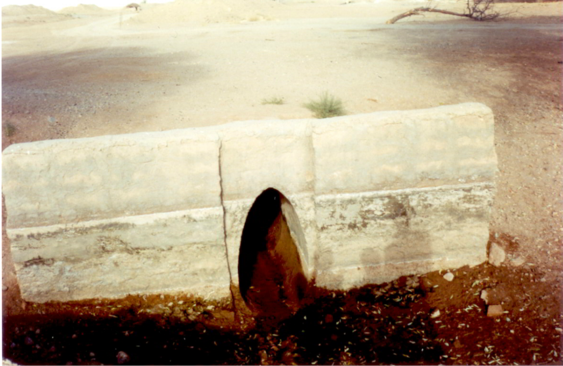
Figure1: Subterranean canal appearance
