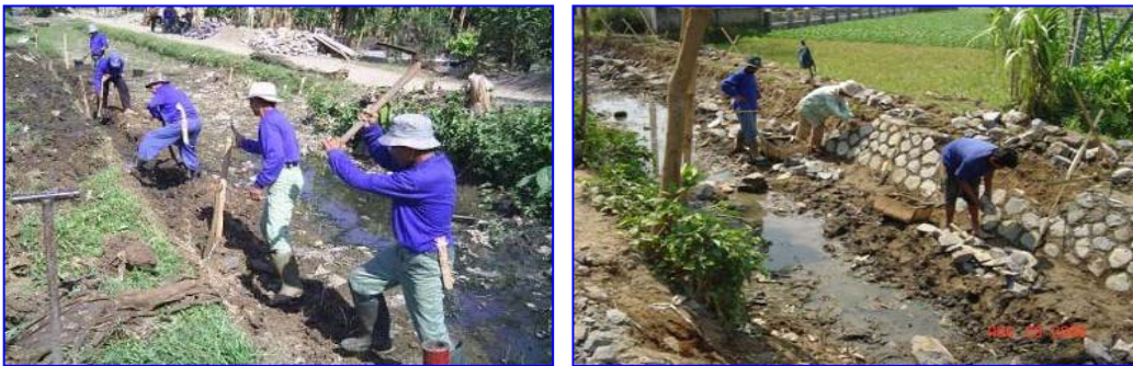
Step VI. Illustration of the mutual work activities for conducting maintenance works, canal improvement and other physical activities of irrigation O&M.
