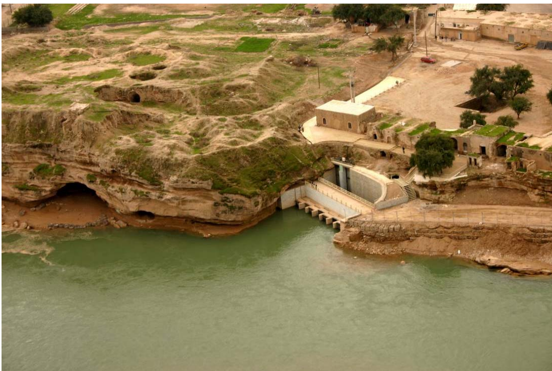
Figure 6. Turn out of Dariun creek
