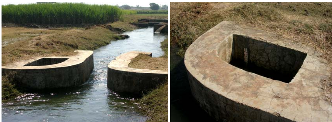
Figure 2. A view of a Standing Wave Flume in operation (left) and a gauge chamber (right)
