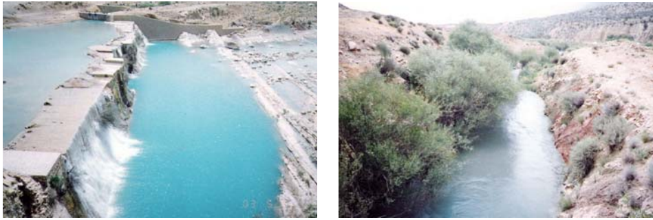
Figure 5 – Bahman Weir with Natural Stilling Basin and A'zam Channel
