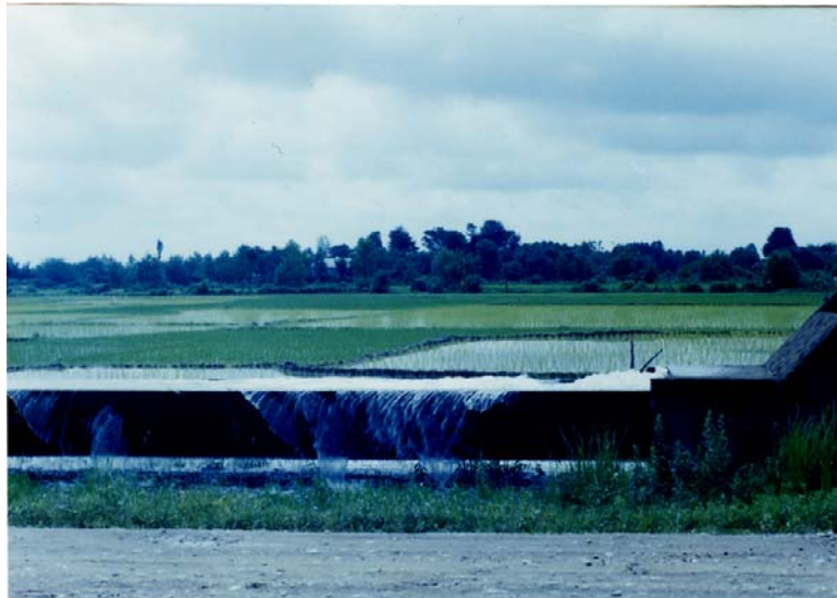
Photograph 4. Creating Blockage in Canal Sections for Getting Needed Water
