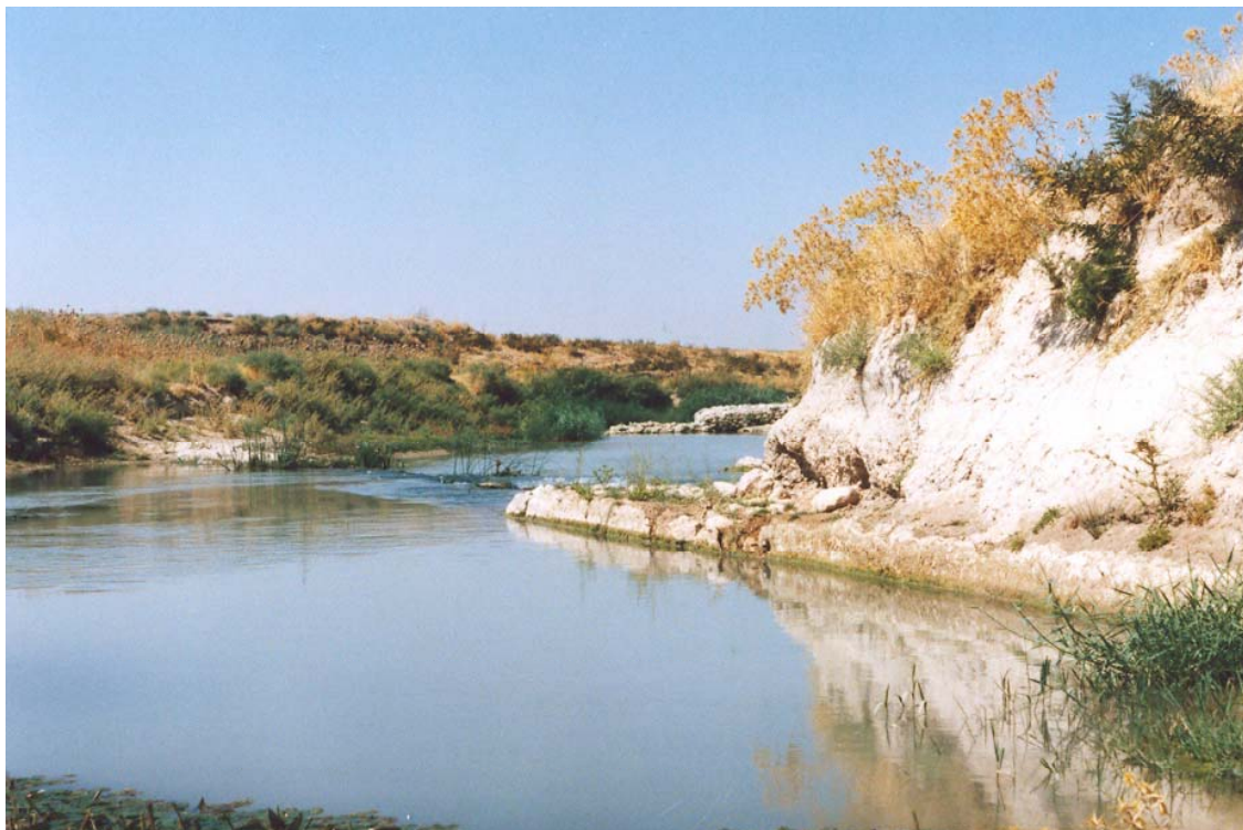
Figure 7. An oblique diversion dam with sarooj plaster on the upstream face.
