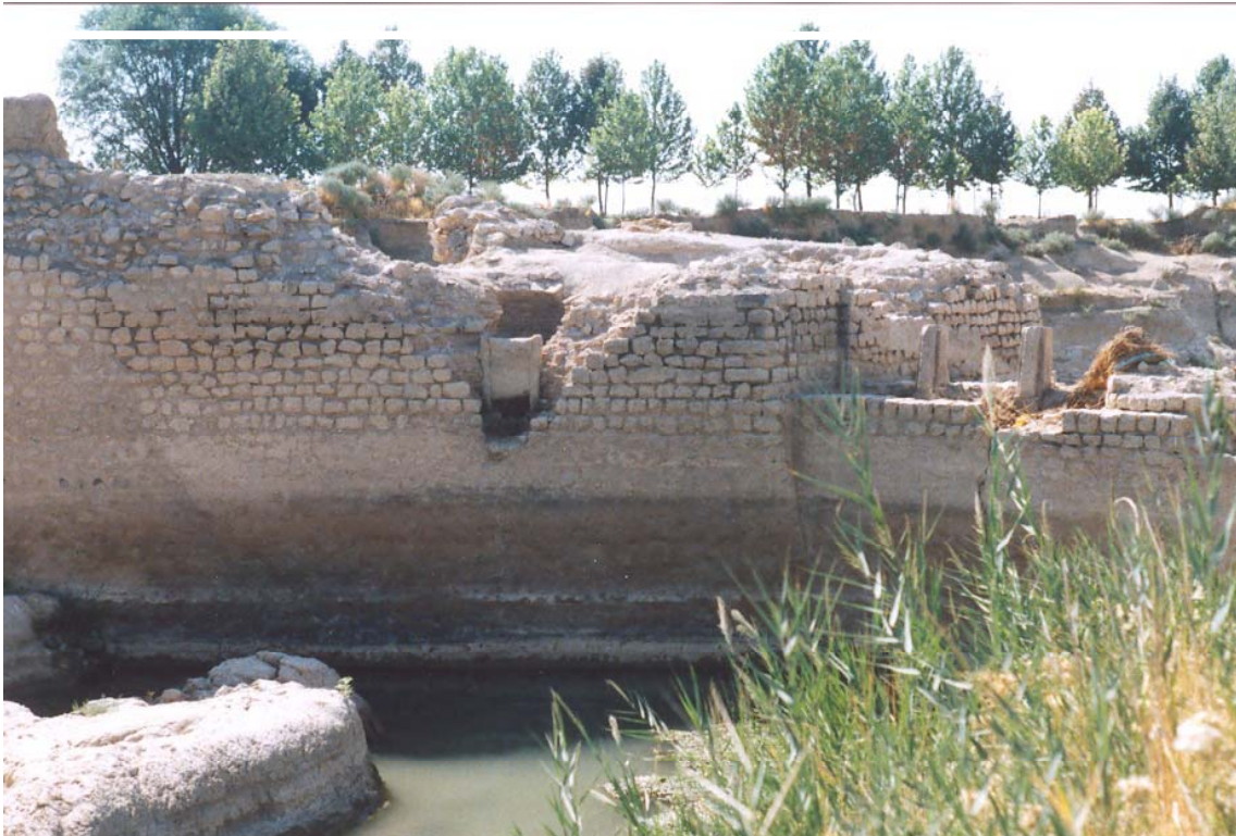
Figure 5. Madabad Diversion Dam on the Sivand River (upstream face).
