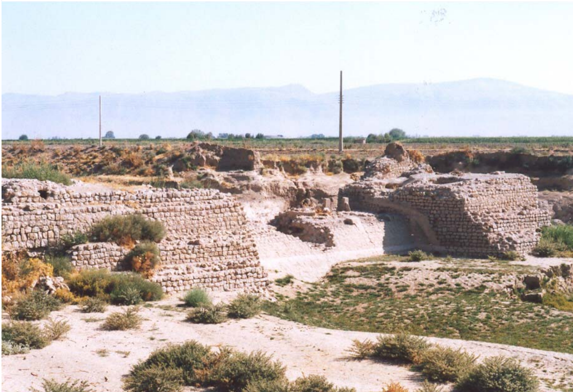
Figure 4. Madabad Diversion Dam on the Sivand River (downstream face).
