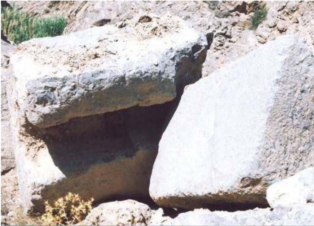
Figure 16. Pieces of U-shape stones making a water conveying small canal downstream of Didegan dam.
