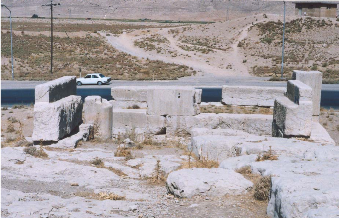
Figure 10. The remainder of Takht-i Tavoos control gate.
