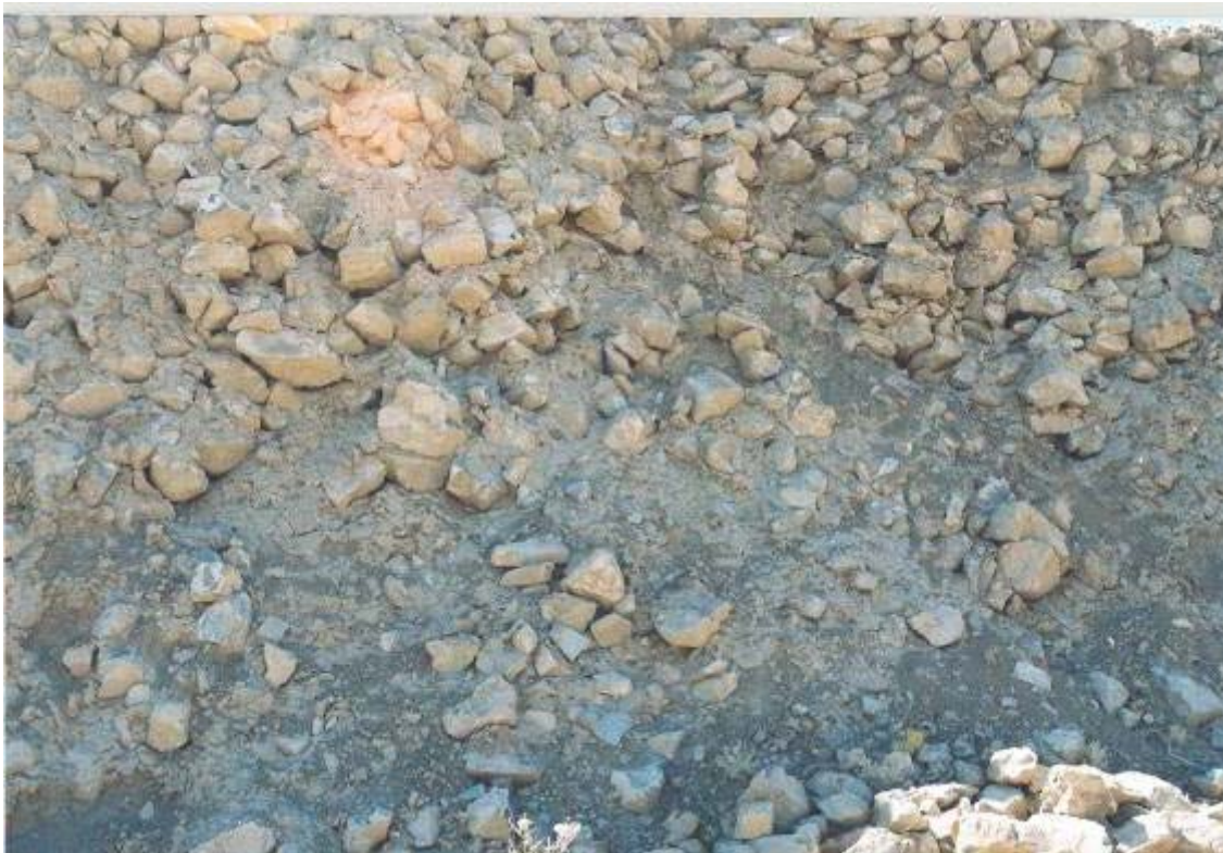
Figure 13. The texture of rock fill parts of Didegan dam.
