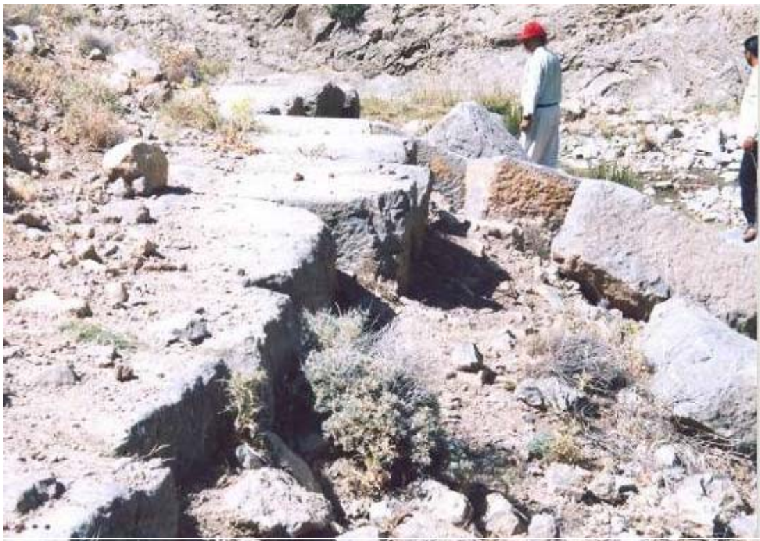
Figure 15. The remaining of stone pavement downstream of Didegan dam. Probably for scour protection.
