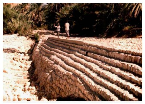
Farmer improved spate irrigation structures in the Hadramawt in Yemen Diversion Weir with a stepped downstream face
