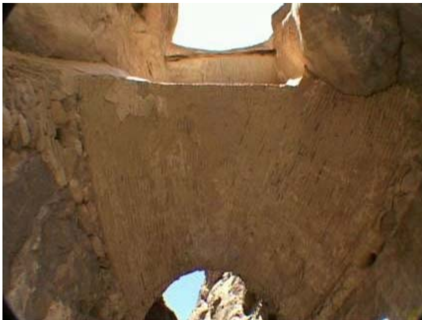
Figure (10). A view of the arch of Abbasi dam from underneath
