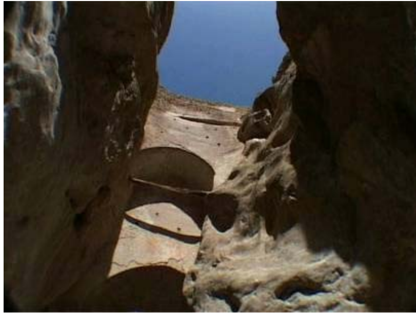
Figure (9). Downstream view of Abbasi retaining dam
