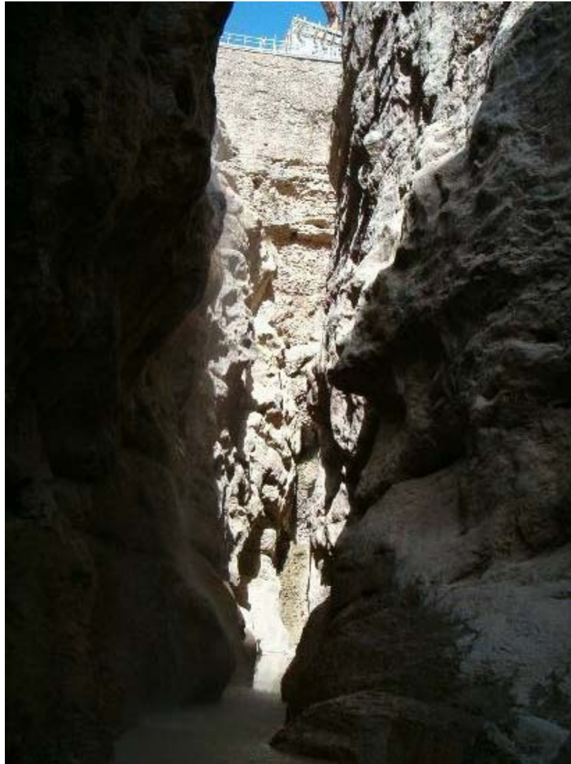
Figure (6). A view 60 m high Kurit dam from the river bed (June 2004) (The left picture is the first picture taken from the downstream river bed due to difficult access to the downstream )
