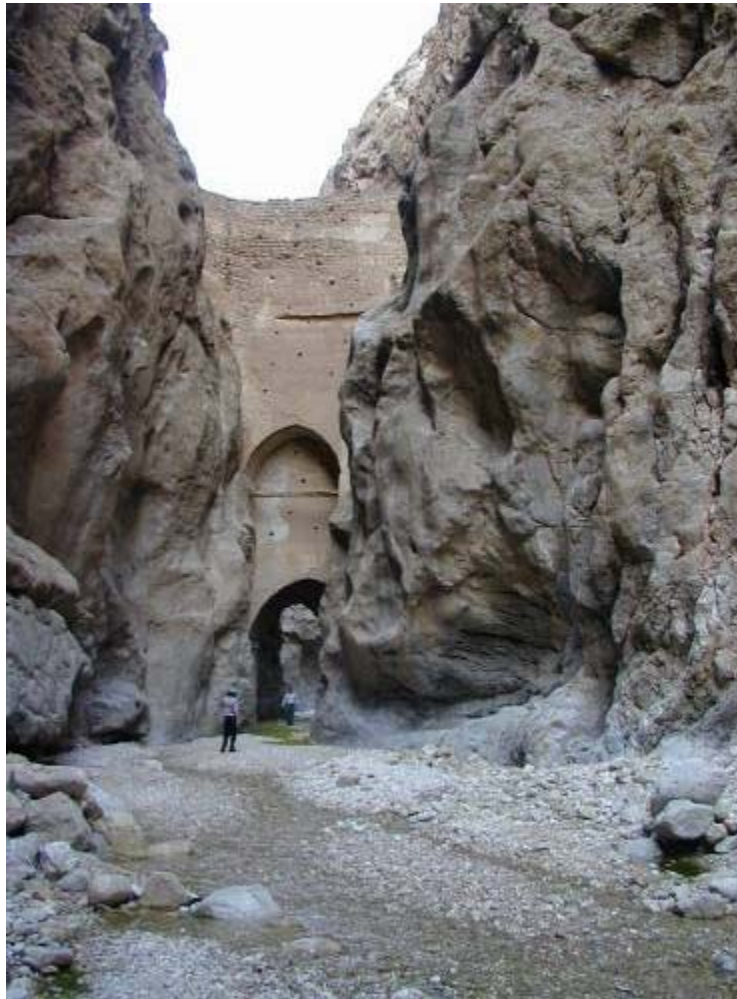
Figure (7) 25 m high Abbasi flood-retarding dam
