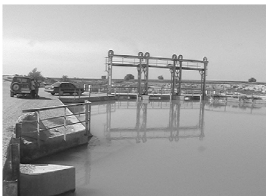
Upstream of diversion dam and canal intakes
