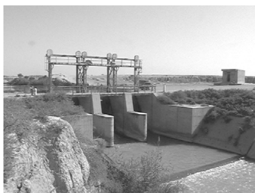
Downstream of diversion dam
