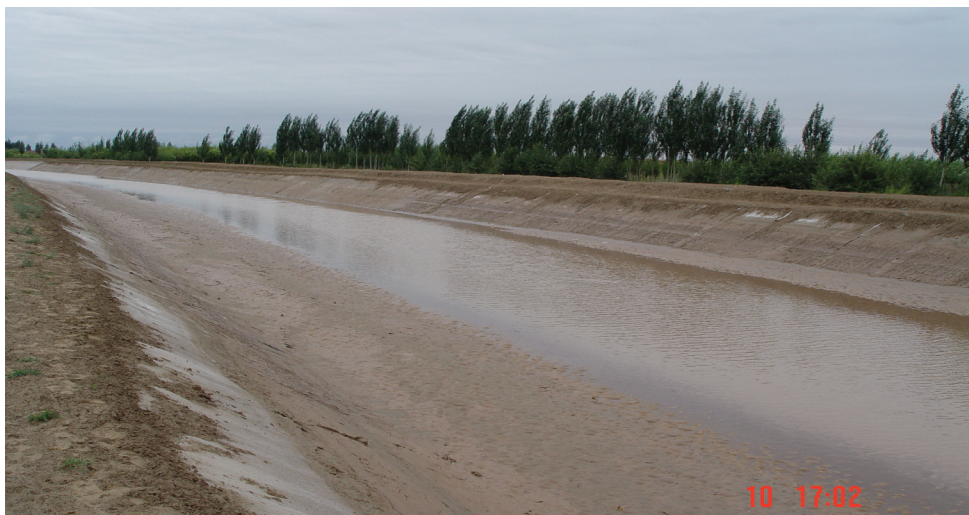
Fig. 6. the stability of side slopes applied with GCL in Yonggang branch canal
