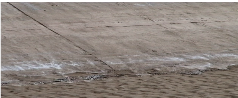
Fig. 4. the canal slopes applied with GCL after the freezing-thawing cycle
