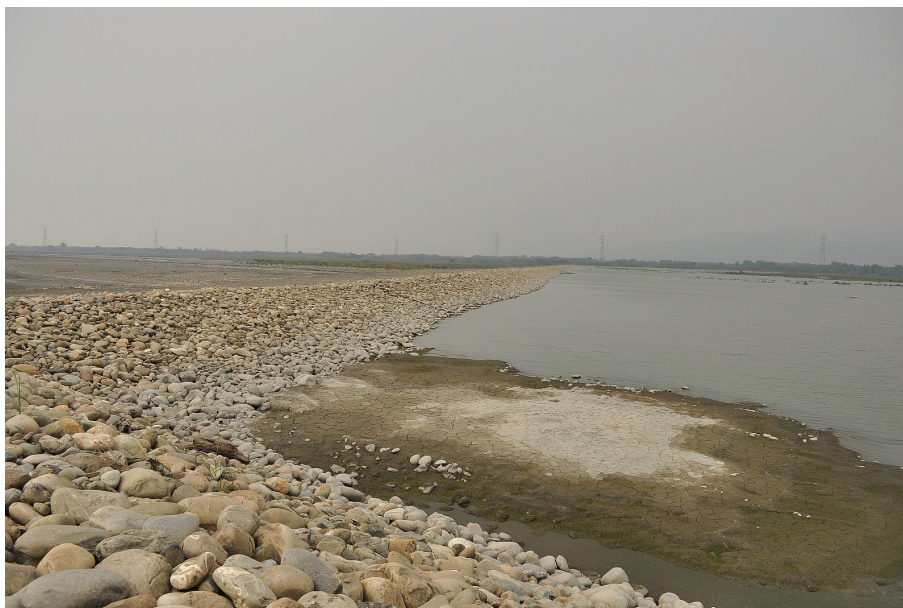
Figure 5. Groundwater recharge in the river channel
