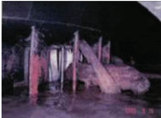
Fig. 4. The turbine was clogged with woody debris (Young and Lai, 2008)
