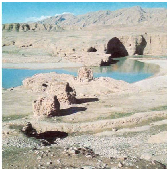
Fig 59 , The ruined structure of Argan Weir on Maroon River.
