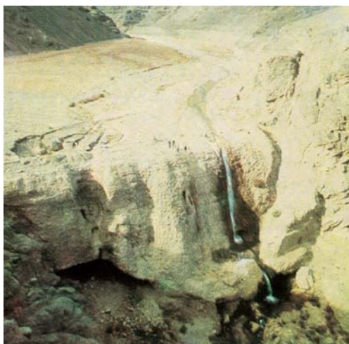
Fig 79 , Qamsar Weir, the reservoir is full of the sediment (age about 400 years)
