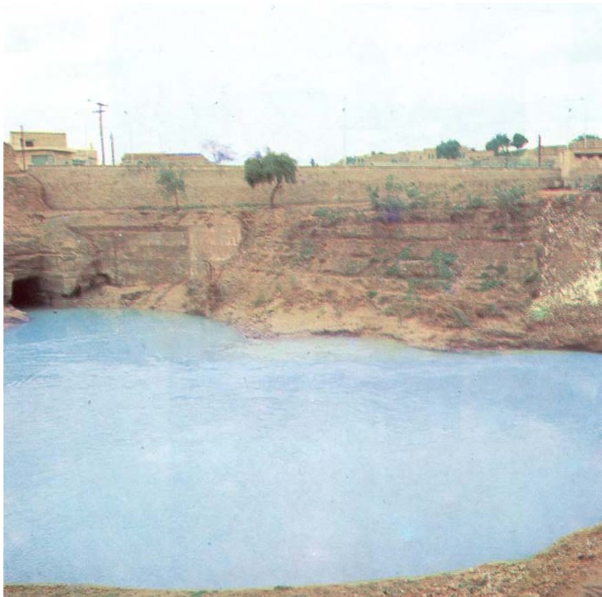
Fig 54 , Gargar Weir in Shoshtar (age about 1700 years). It is still under operation
