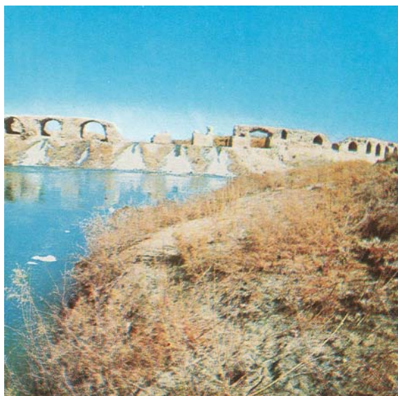
Fig 68 , Tilikan Weir Bridge on Kor River (water mills)
