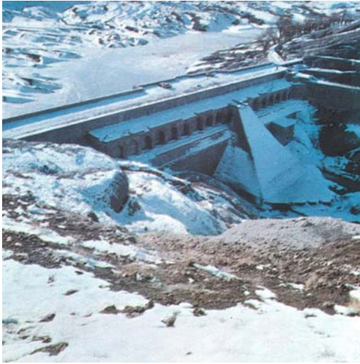
Fig 85 , Fariman Weir, view from downstream
