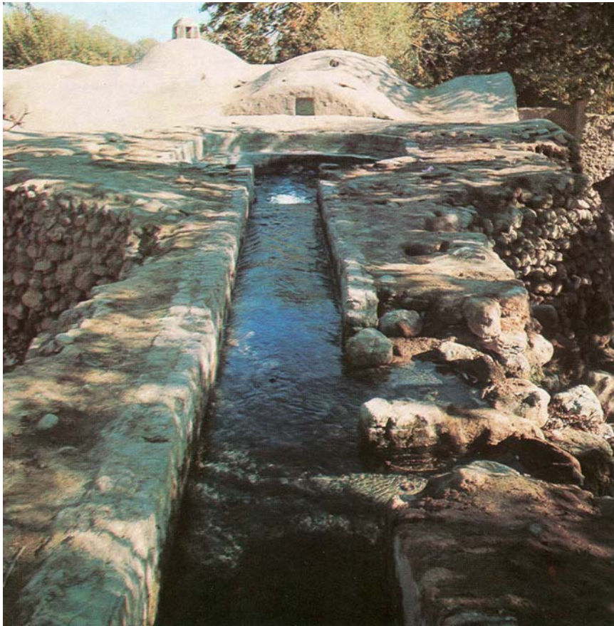
Fig 45, Here is Sohrab Canal which belongs to one of the mills in Feen Gardan in Kashan. The spillway and diverting channel are shown in the right side and the roof of the mill in the rear.
