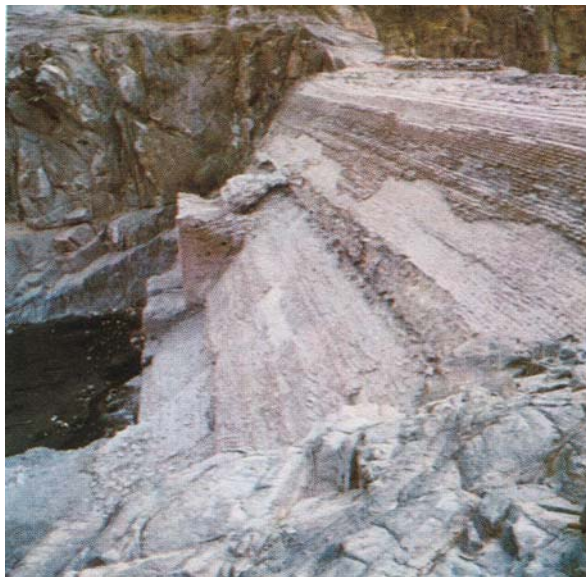
Fig 90 , Golestan Weir, view from downstream
