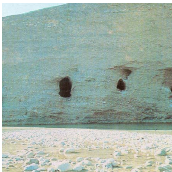
Fig 60 , Water intake at the upstream of Argan Weir. It was constructed like qanat.
