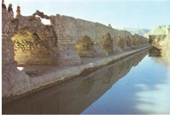
Fig 64 , Amir Weir Bridge, view from upstream
