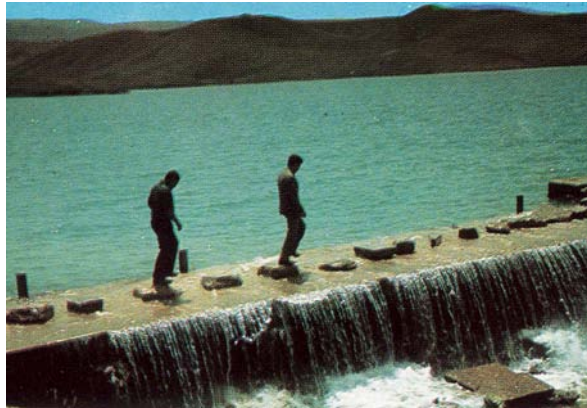
Fig 105, Fariman spillway located at the left bank
