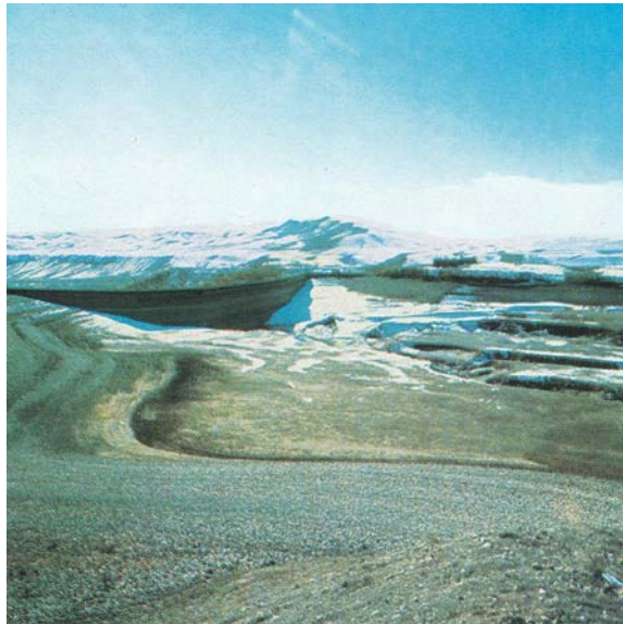
Fig 88 , Salami Weir, view from upstream
