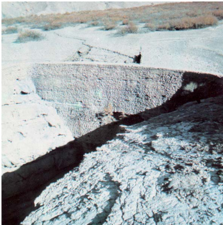
Fig 86 , Koreit Dam in Tabas, it is an arch dam, the height is more than 100 meters. The reservoir is full of sediment (age about 400 years)
