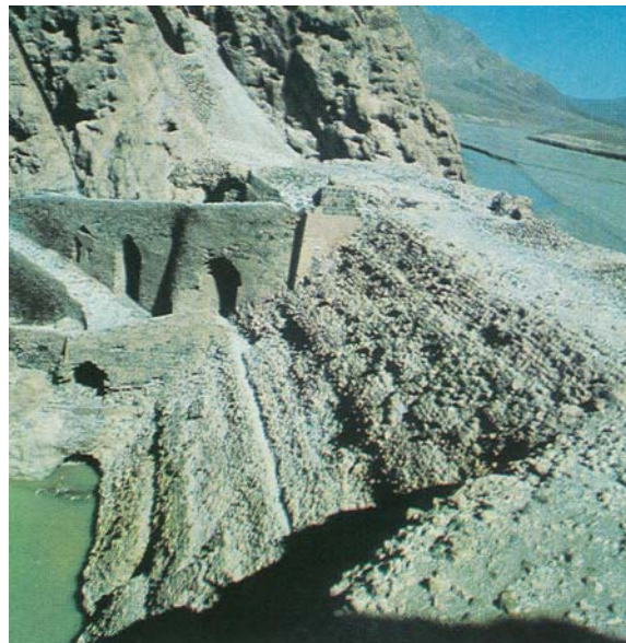
Fig 73 , Saveh Weir, view from upstream (age about 700 years)
