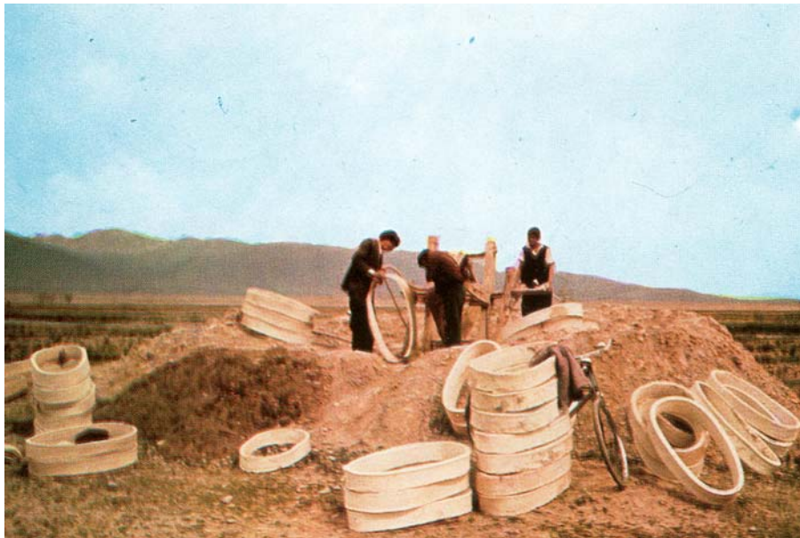
Figure 156, Some ceramic rings for lining the gallery in crumbling soft lands.
