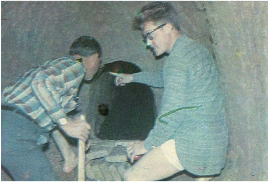
Figure 155, This is a cross section of a Qanat's gallery in the town of Sabzevar. The Qanat is being used for the modern domestic water network by putting pipes in it.
