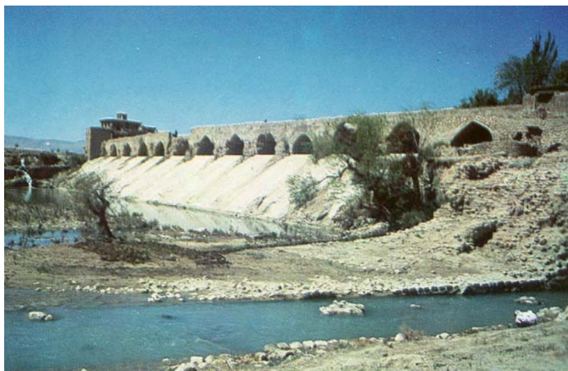
Fig 107 , Natural stilling basin of Amir Weir
