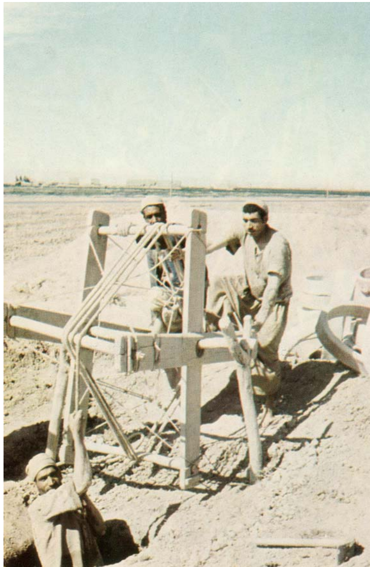
Figure 161, A windlass for sending up and down the workers and debris.
