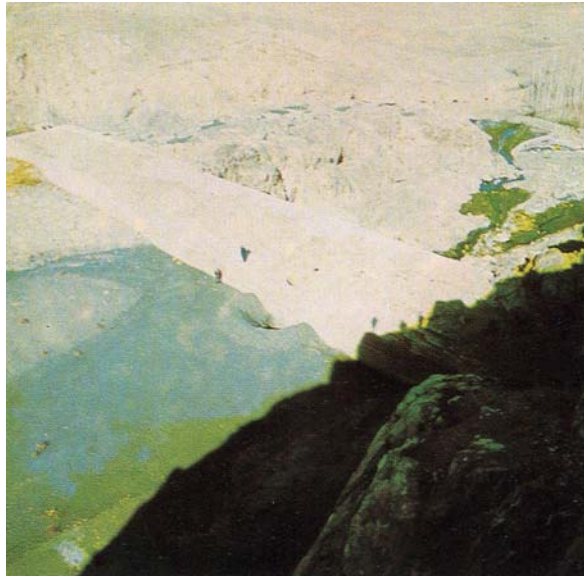
Fig 89 , Golestan Weir in north of Meshad, the reservoir is full of sediment (age about 300 years)
