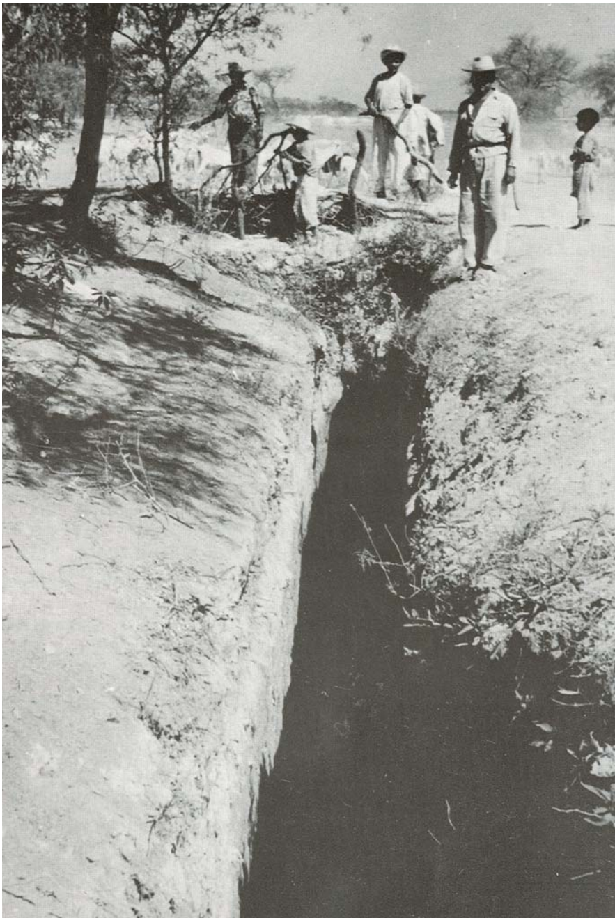
Figure 174 , The shafts of a Qanat in Mexico. The Mexican natives call the shafts Lumbreras which means chimney. They also call the tunnel Galeria Filtrante which means infiltrated gallery.
